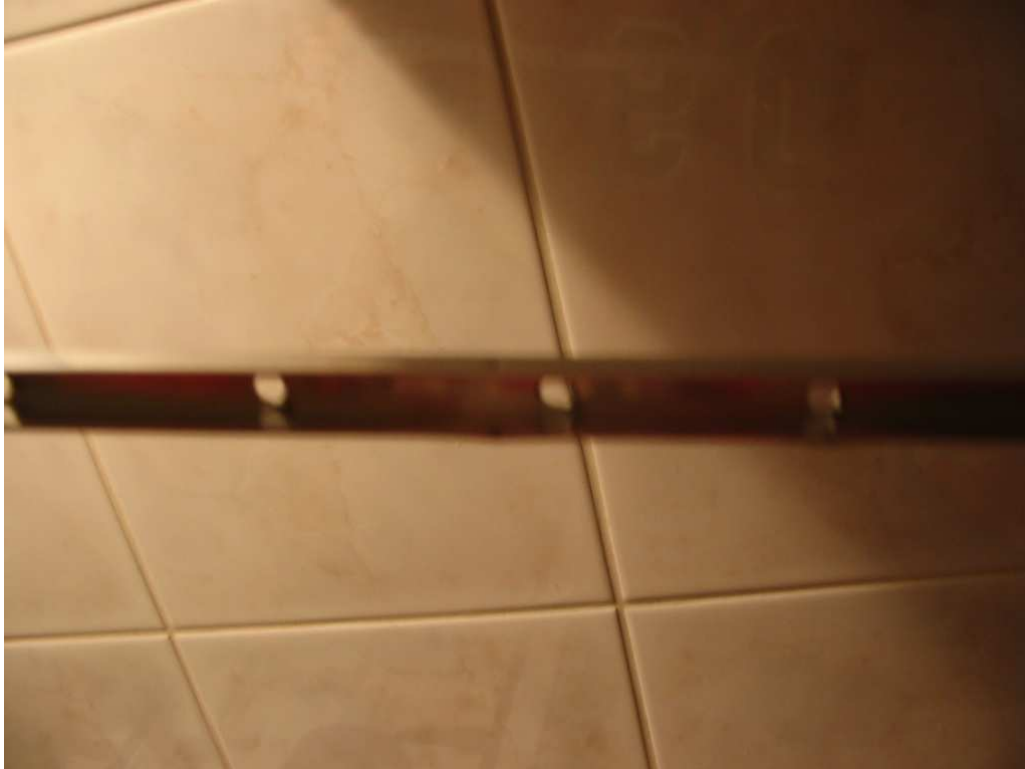
Image 14: Drilled holes in aluminum U-frame
